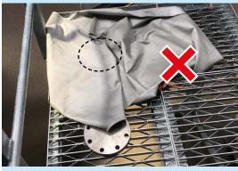
A hole with its cover removed is not visible beneath this cloth. A potential safety hazard.
